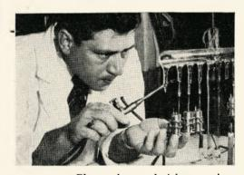
▲Electronics technician seals new and rugged, SRI-designed klystron tube on vacuum pump.
