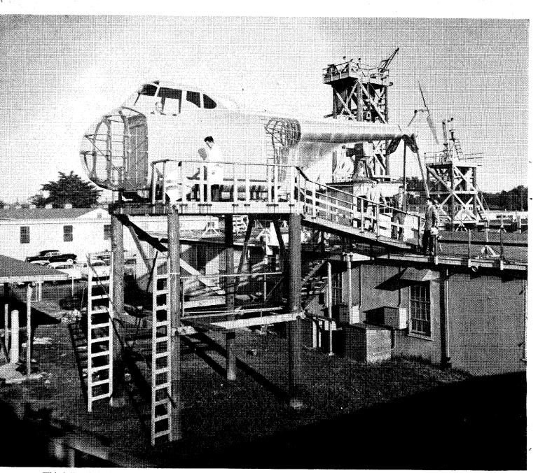
This full-scale helicopter mock-up is used for testing flush-mounted radio antennas. Below: SRI director Jesse E. Hobson.
